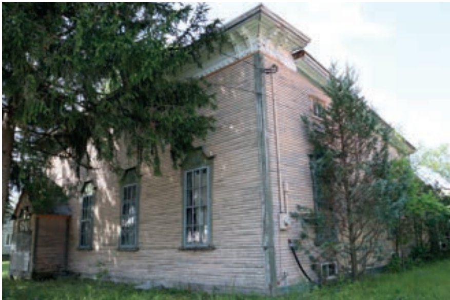
Temperance Hall (1889) ; 9, rue Colville, Howick
