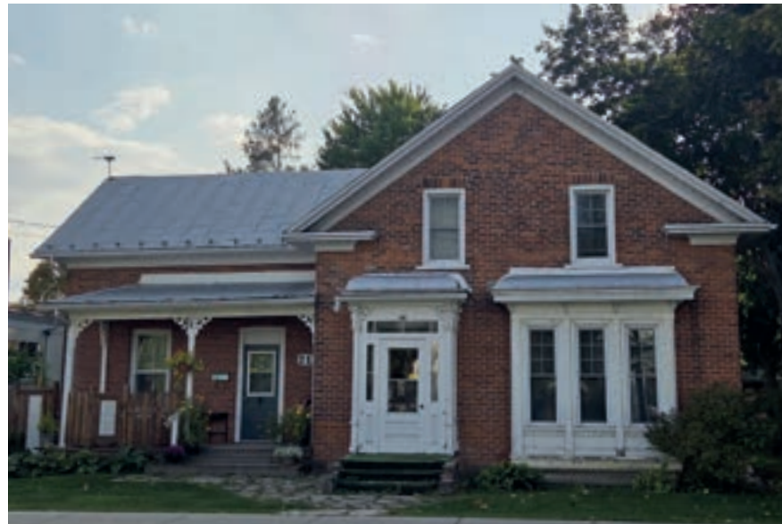
21, rue Church, Ormstown
