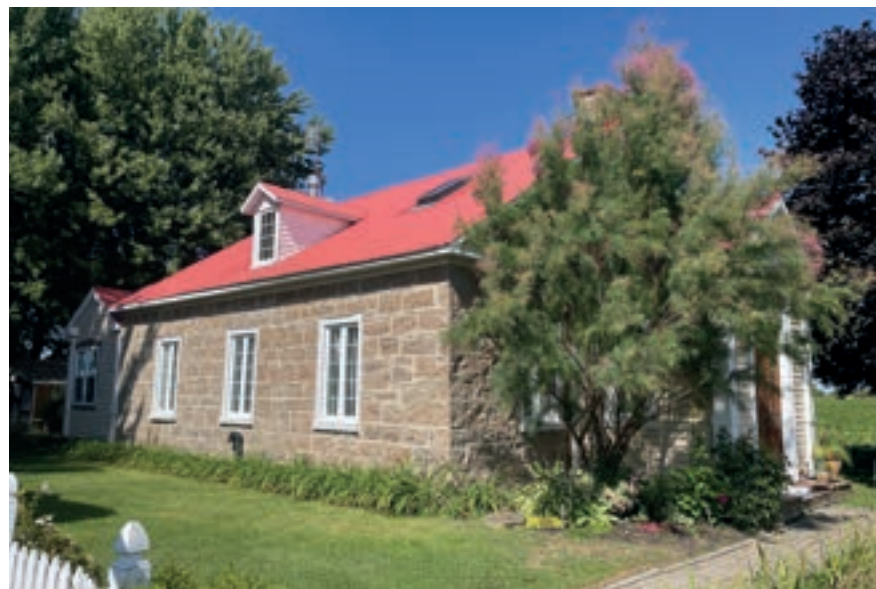
Stone School (1840) ; 2435, chemin Lower Concession
